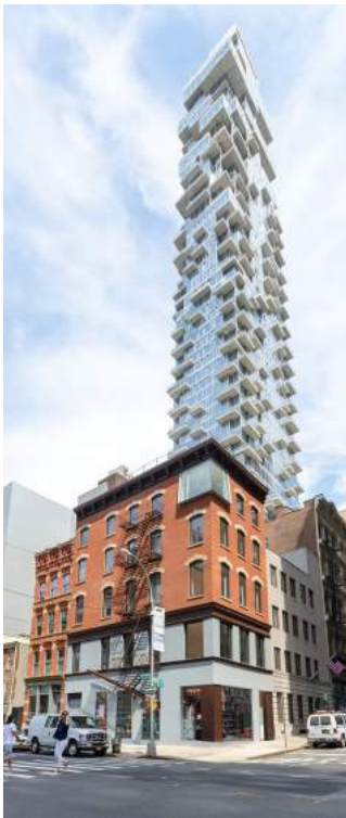
Exterior West Broadway Facade
